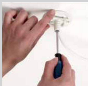
Fix mounting plate(s) to the surface/ BESA box, using the fixing template supplied if required.
